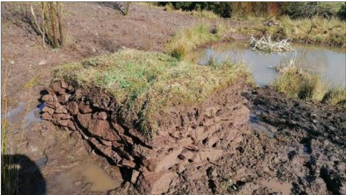
Plate 4.7 An example of a recent biodiversity/wetland pond creation in Watergrasshill, Co. Cork showing installation of a dry-stone, grass-capped hibernacula in foreground (credit: Triturus)
